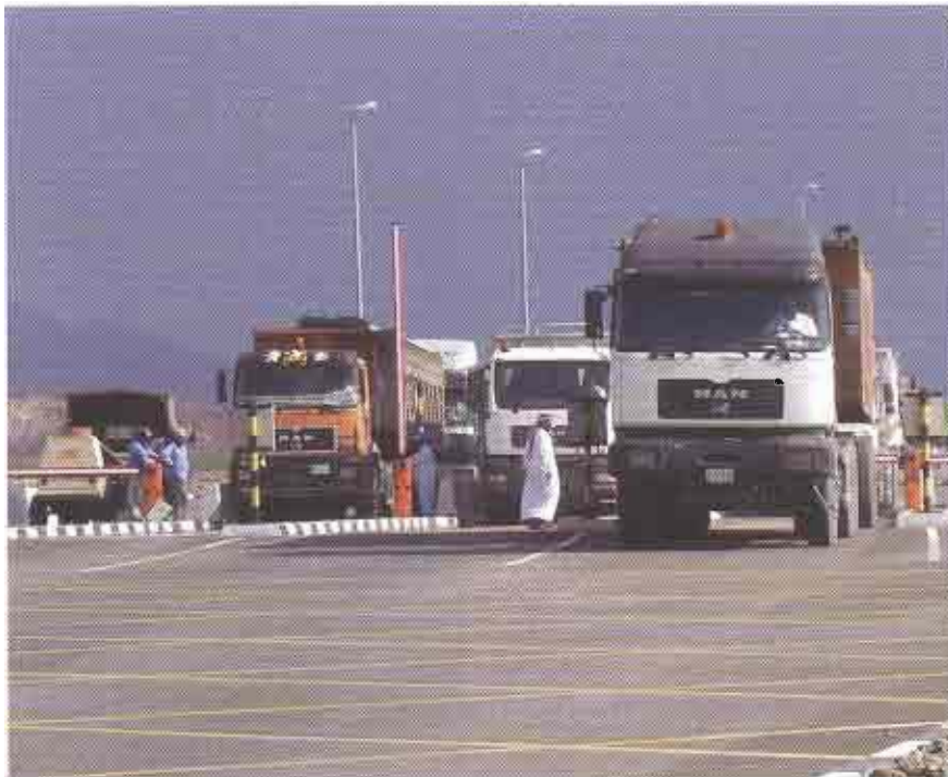
Central Weighing's Supaweigh system in Fujairah has been designed to cope with 110-tonne gross loads
